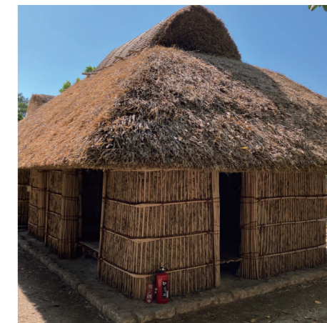
茅葺屋根補修
